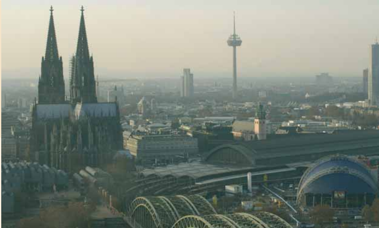
The flow of energy is optimized around the city of Cologne by a sophisticated integrated network.
