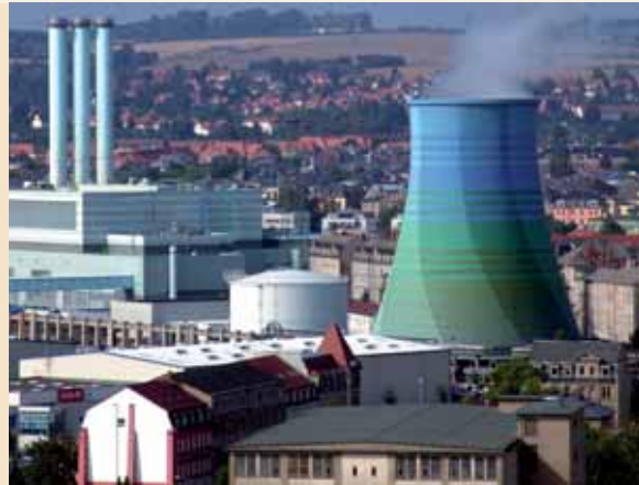
Modern DREWAG CHP plant.
