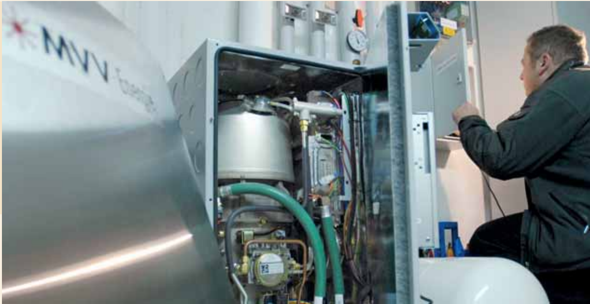
The electricity-generating heater called “WhisperGen” consists of a Stirling motor and heat exchangers. These components are integrated into the heat and power supply system in a house, and monitored remotely using cutting-edge technology.
